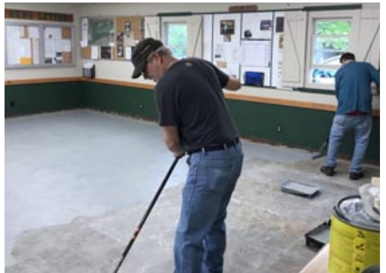
Range Construction painting clubhouse floor.
