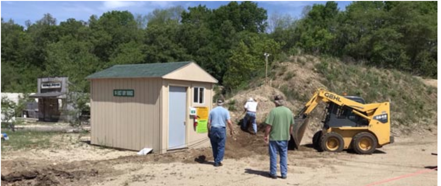
Range Construction installing the new camera system.
