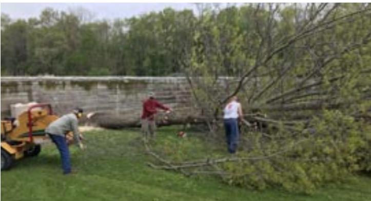
Range Construction removing trees for the new safety wall.
